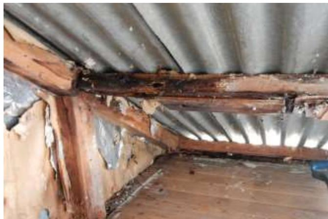
Above: The rotten purlin. Note the rusted nail not attached to any timber
