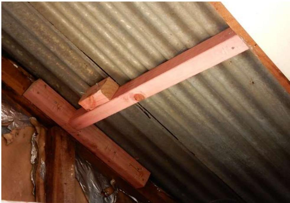
Above: The combined purlin & rafter brace in position. Note the extra block where the old lead-head nail came through the roof
