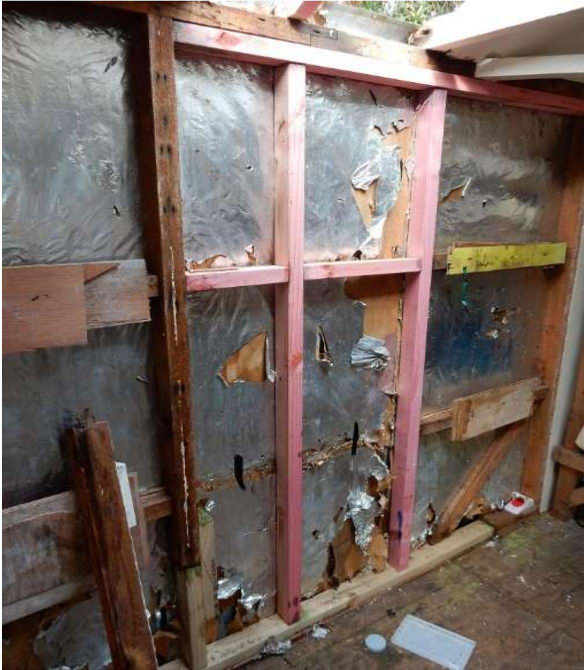
Above: In with the new bottom & top plates, studs & 2 of the 4 dwangs
