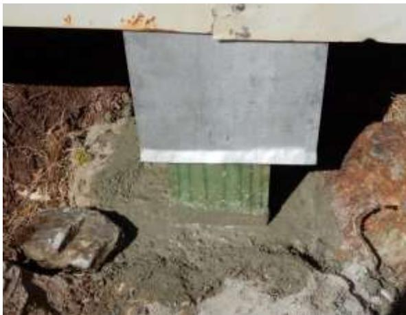
Above: New flashing to protect the new bearer & top of pile
